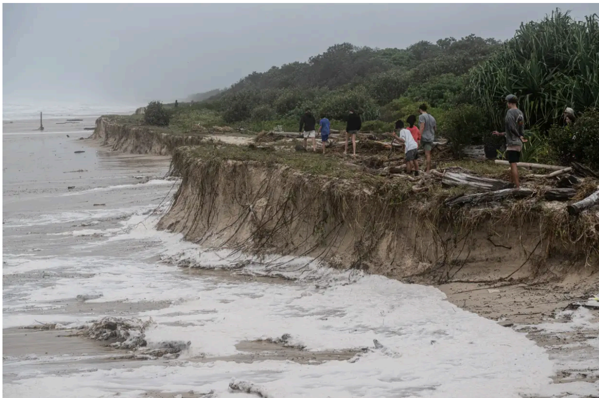
Cyclone Alfred has already caused severe beach erosion. Nick Moir
